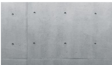
Concrete wall (with gypsum board substrate)
